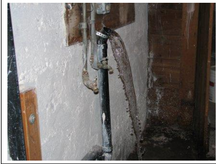
As the bathtub drained on the second floor, water started to exit out the cloths washer drain in the basement. The sewer line had some issues.
