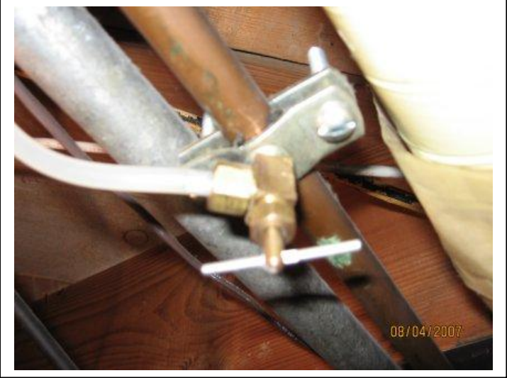
If you see this in your house, replace with a t fitting and a real shutoff valve. New homeowner did not. Water damage in basement six months later. When they go, they go!
